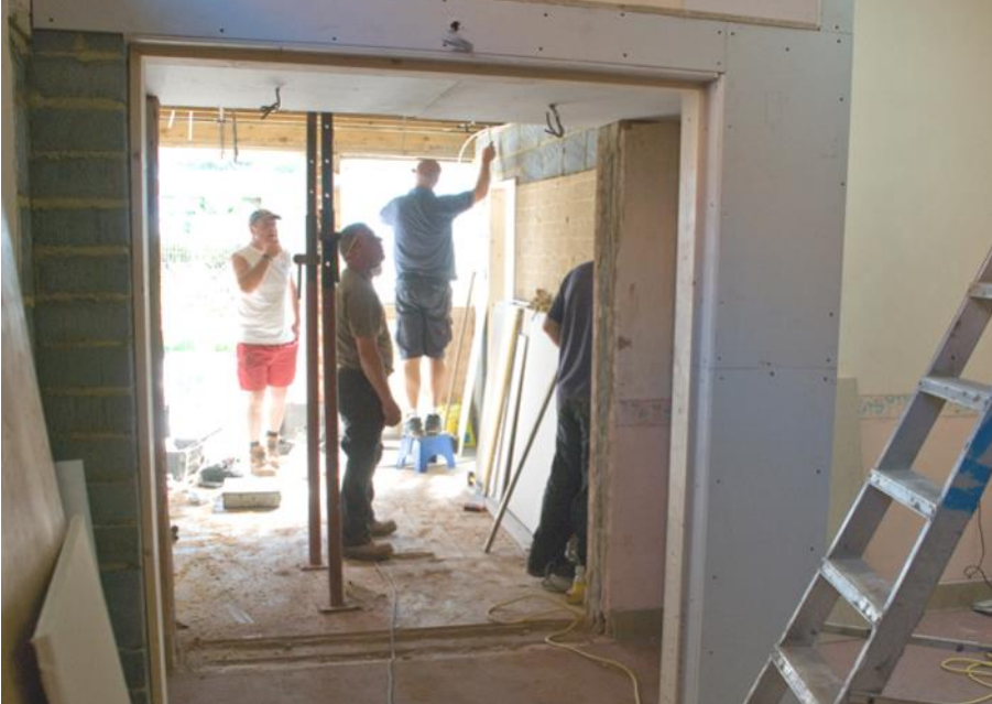
Looking from the newly constructed Cornwall room through the demolished wall to the Entrance Hall to outside.
